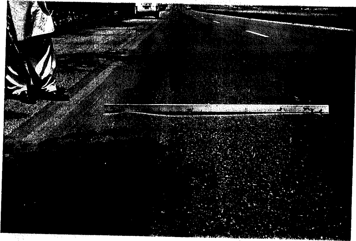
Plate 7-18-3 Severe rutting being observed and shoving along the side of rut is clearly visible on Old Carriageway.
